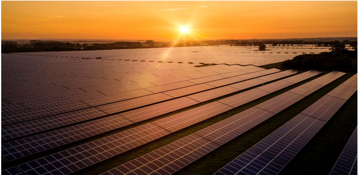
Image 3.1 Typical Fixed South Facing PV Arrays
